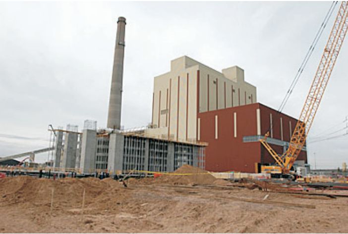
Weston 4 unit under construction near Wausau, Wisconsin
