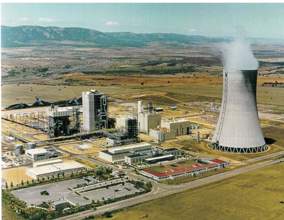
A commercially operating gasification plant in Spain.
