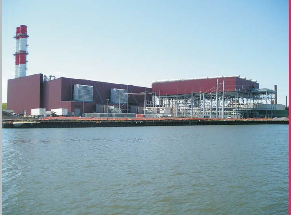
Astoria from ConEd looking southwest.
